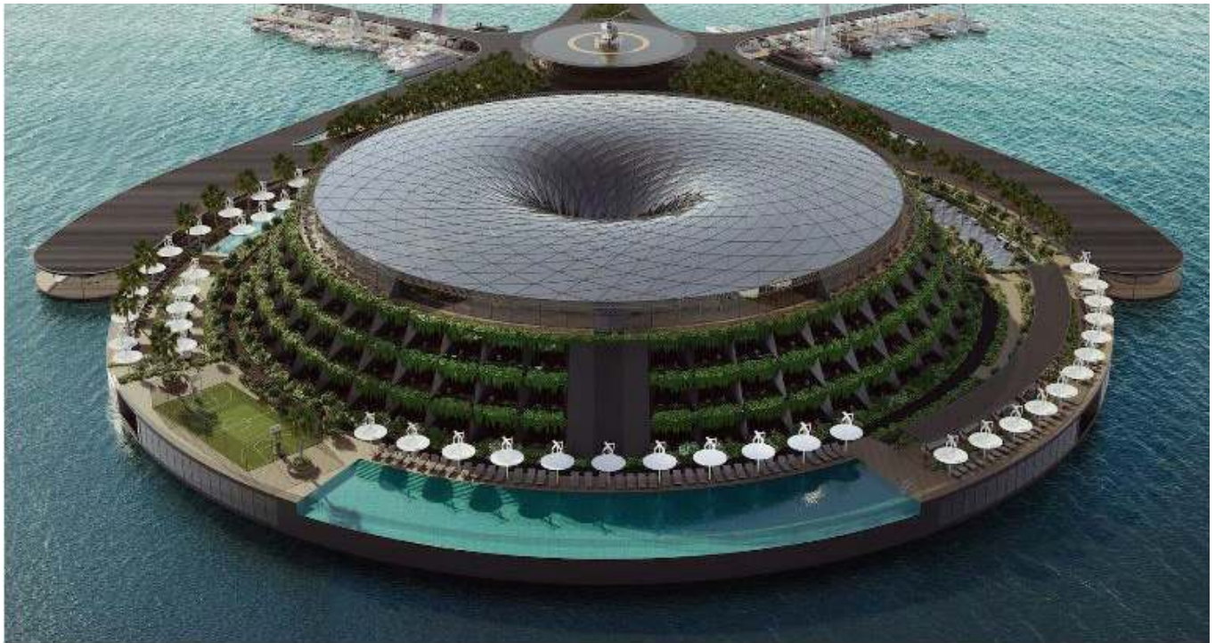
Here's what to expect from Qatar's upcoming floating hotel project (Photo: Courtesy of Hayri Atak Architectural Design Studio)
