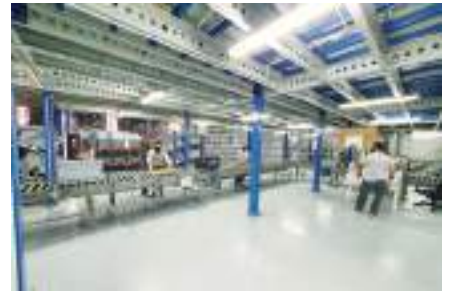
The NET Fulfillment Center rebuilt & back on track
