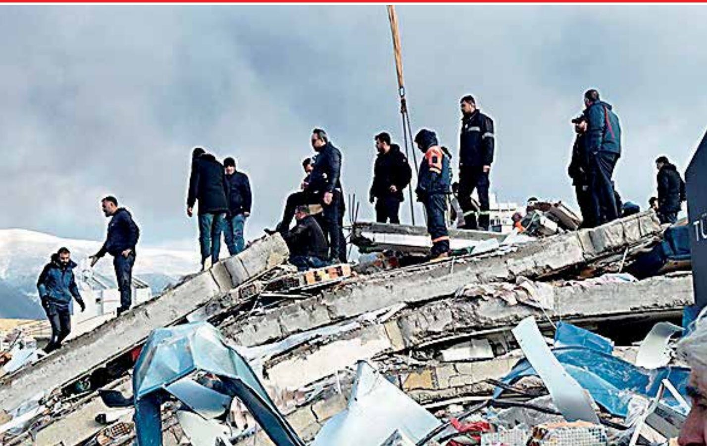
Search for survivors in the rubble of a destroyed building in Iskenderun, Turkey - Source: CTK/Alamy Stock Photo
