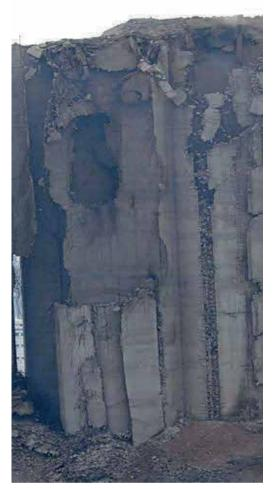
A left part of the silos damaged during the Augus silos collapses, 2 years after blast
